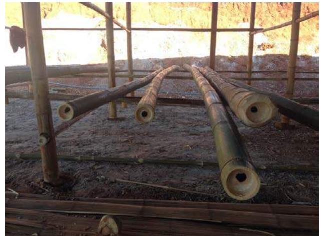
Drilling of Bamboo nodes for full saturation of Borax solution in bamboo
