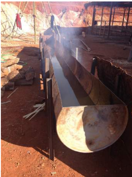
Solution heating in tank
